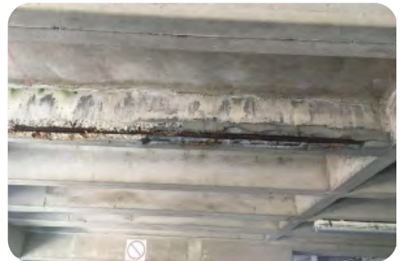
Exposed Rebar
